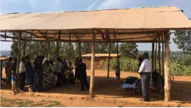
(Above) Like many churches in Rwanda, this church that was started by one of our graduates faithfully met in a facility with no walls.
